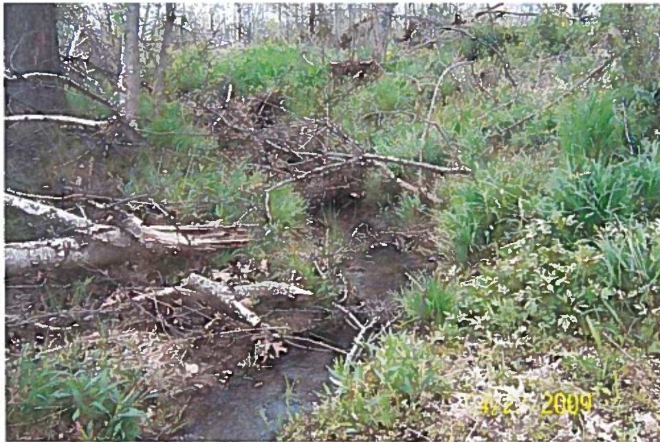
Station 154+49, Sheet R15, Intermittent, RBP score 110/poor
